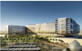
Data Center for Prince Mohammed Medical City - KSA
