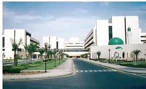
Data Center for King Fahad Medical City - KSA
